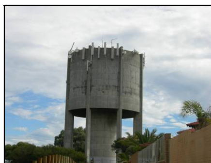
Tank with Communications Equipment Owned by Others
