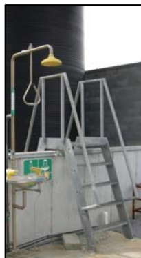
Example of Steps for Accessing a High Walled Bund
