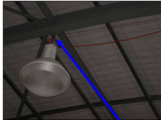
Fitting can be lowered to ground level
