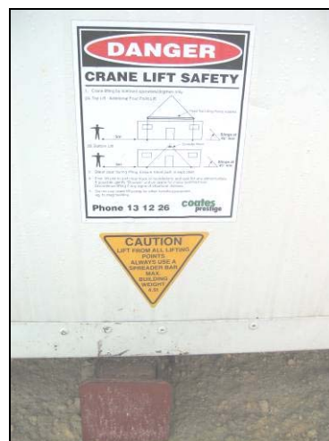
Example of a lifting lug at the bottom of a transportable building
