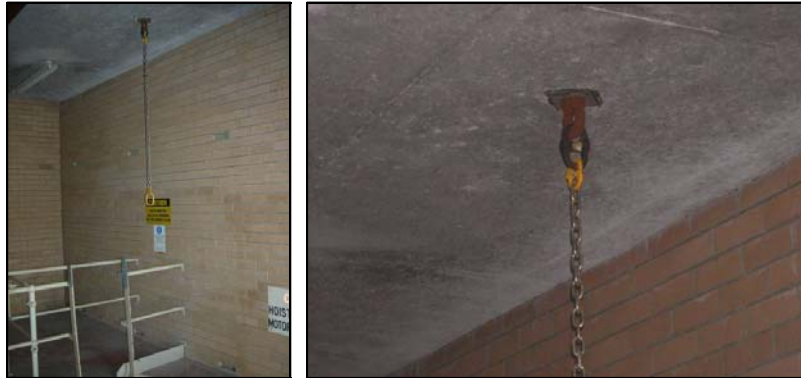
Example of an Anchor Point and Chain for Winch Attachment
