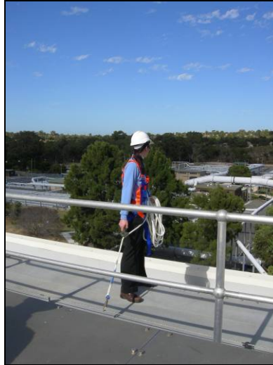
Static Line and Rope Grab Roof at Beenup Waste Water Treatment Plant
