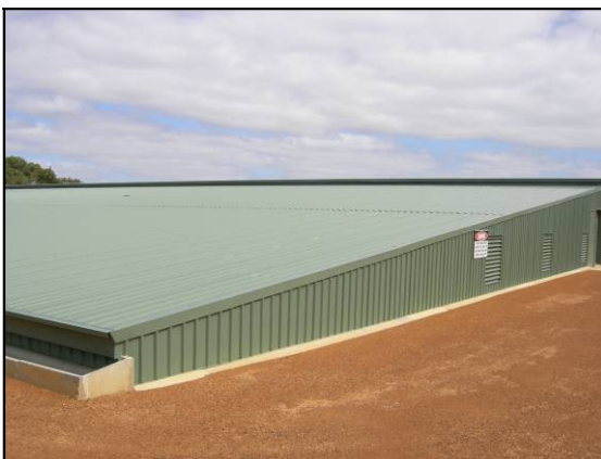
Typical Reservoir Roof
