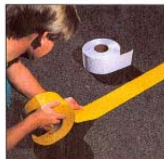
Use pavement Marking Tape to temporarily redirect traffic on highways or around construction sites, or to temporarily mark driveways and parking lots.
